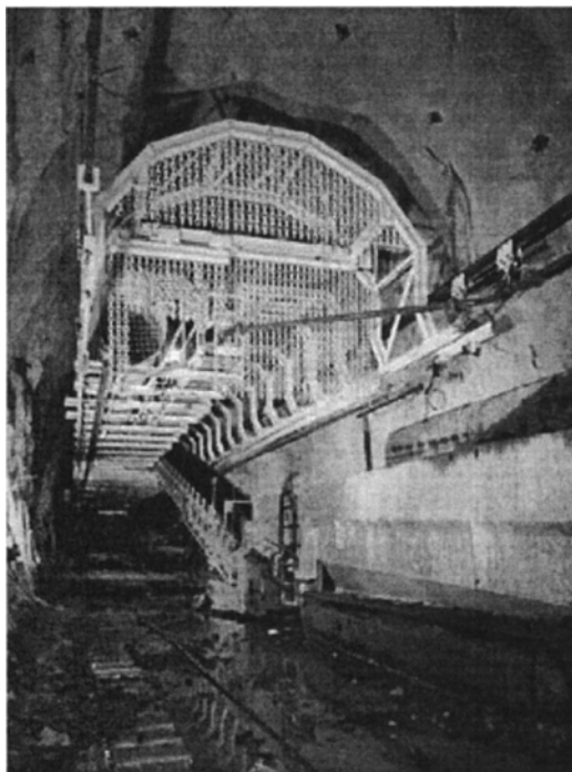
Fig. 8. View of equipment from face of tunnel—rock crusher, inclined conveyor belt hanging chain for fly rock protection
