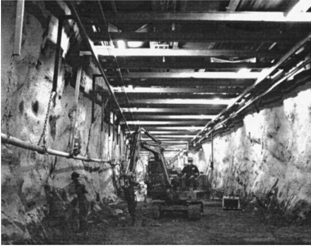
Fig. 10. Invert excavation, using hydraulic hammer mounted on small excavator boom, taking place underneath suspended excavation services platform
