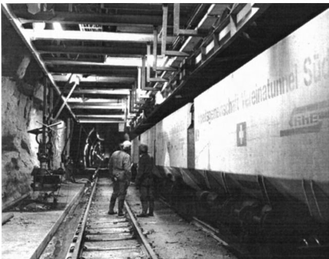
Fig. 11. Loading bridge area with muck transfer from suspended excavation services platform conveyor to muck train
